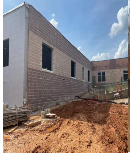
Split Face Block Completed at SE area of building
