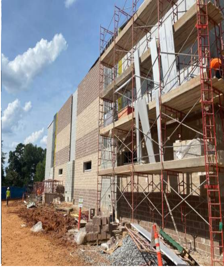
Split Face Block Installation at Perimeter
