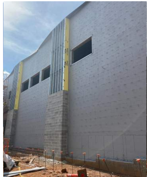
Framing at pilasters
